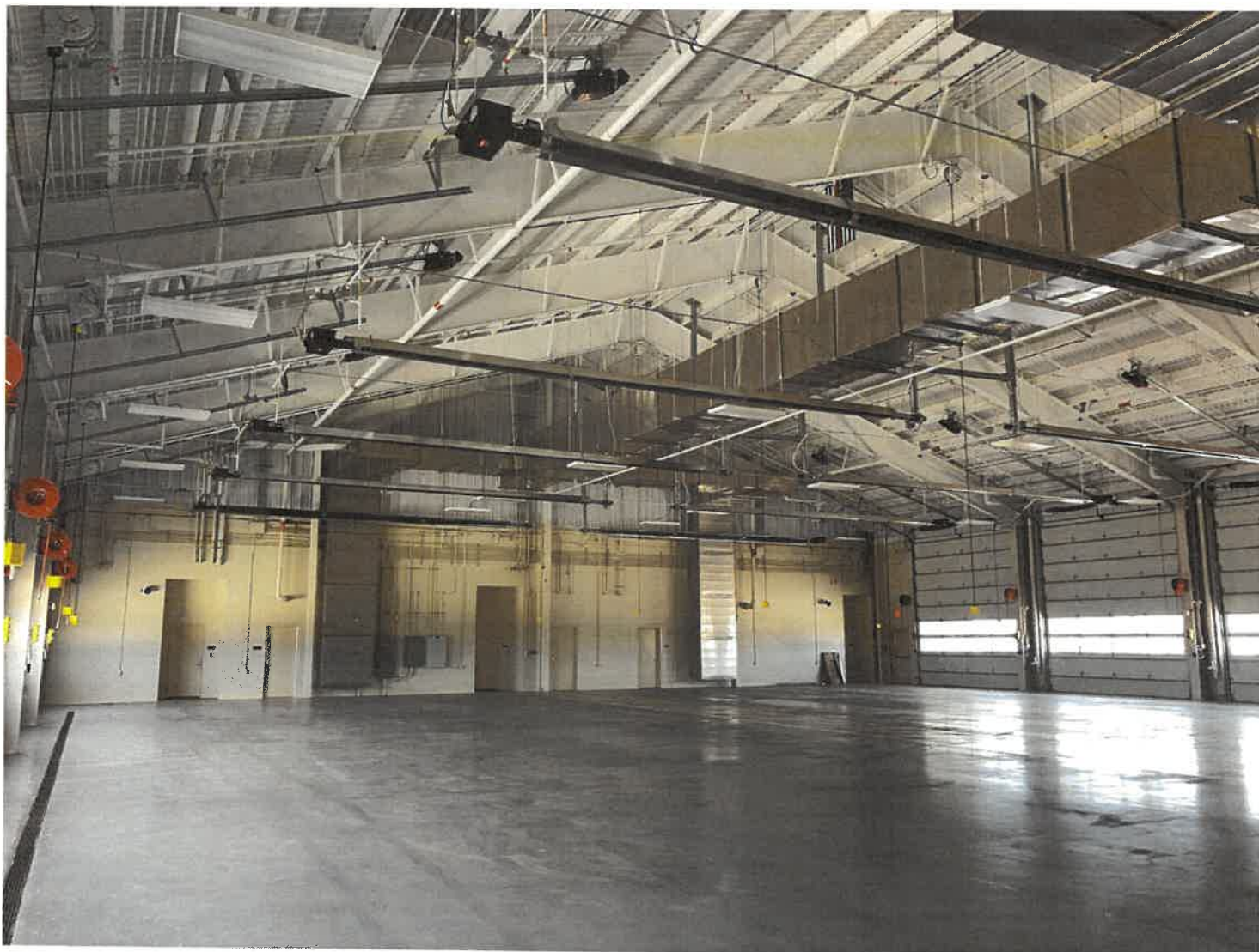
Eglin AFB, Fire Station #1, PEMB Bay
