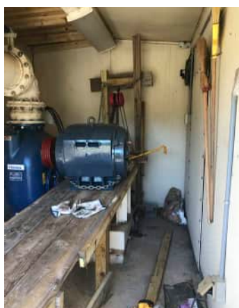
Replaced the 100-horsepower (hp) motor for pump 3 at the Lloyd Street lift station.
