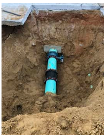
Replaced 12 inch distribution valve at the RIBs.
