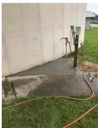
Installed reuse hose spigot for Digester 2.
