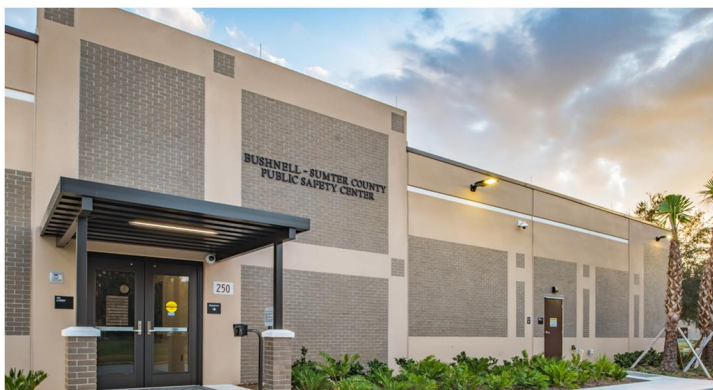
SUMTER COUNTY PUBLIC SAFETY BUILDINGS
