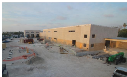
Transportation & Internal Services Facility Live Web Cam
