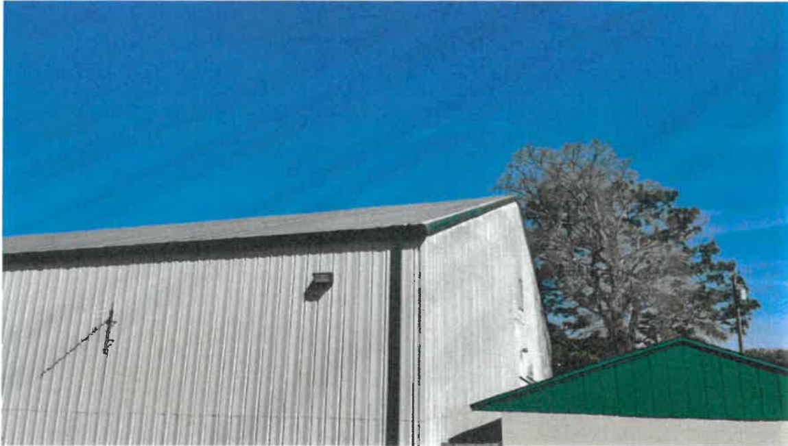
Overview of roof system
