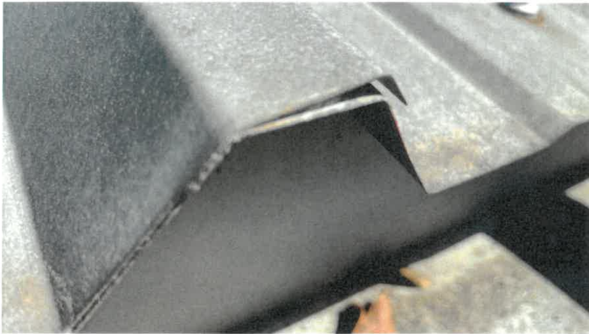
Overview of gutter and metal edge overlay
