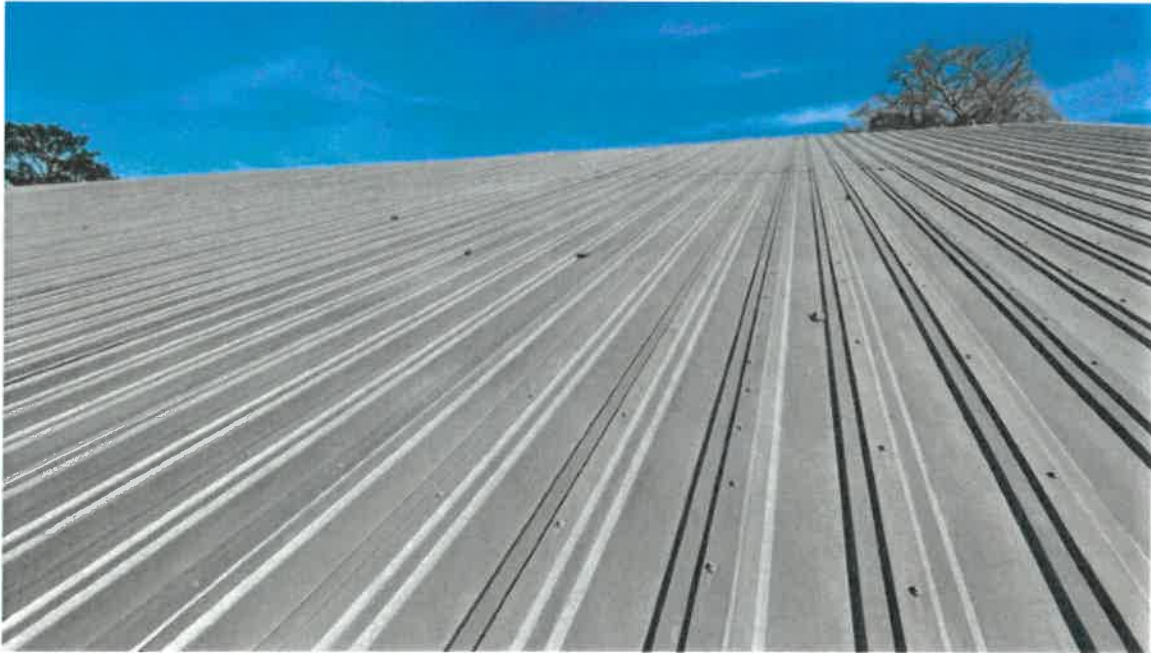
Overview of roof system
