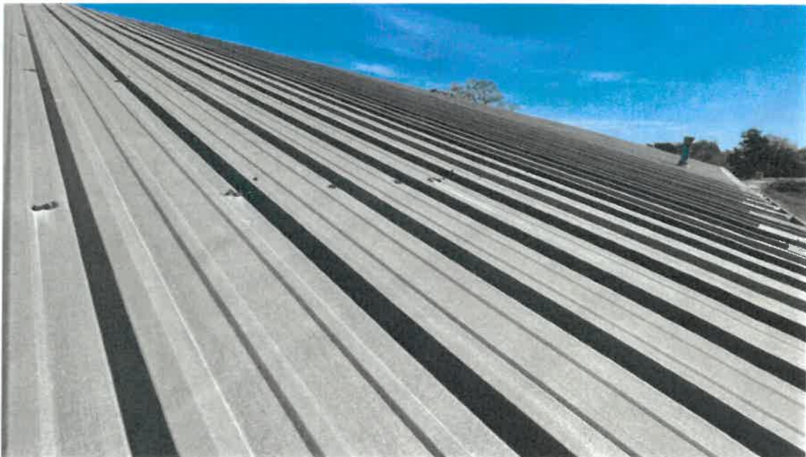
Overview of roof system
