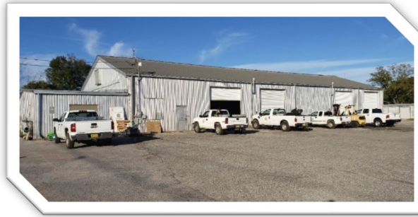
Figure 3. DPS Complex Garage
