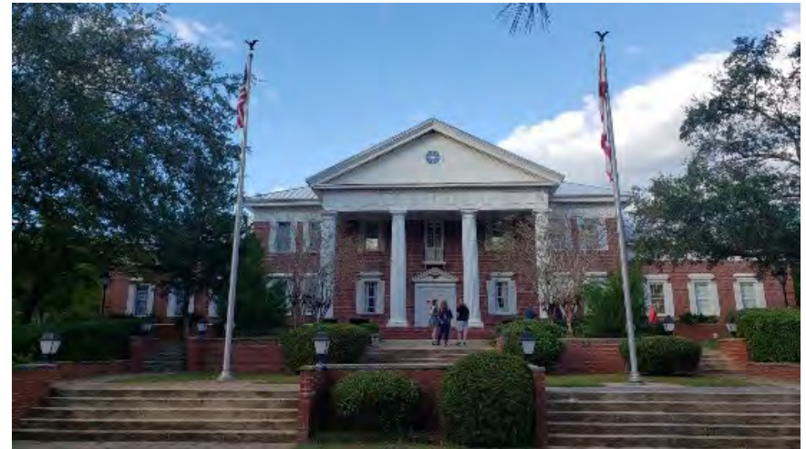
Photo of the Northwest Florida State College Robert L.F. Sikes Center building.
