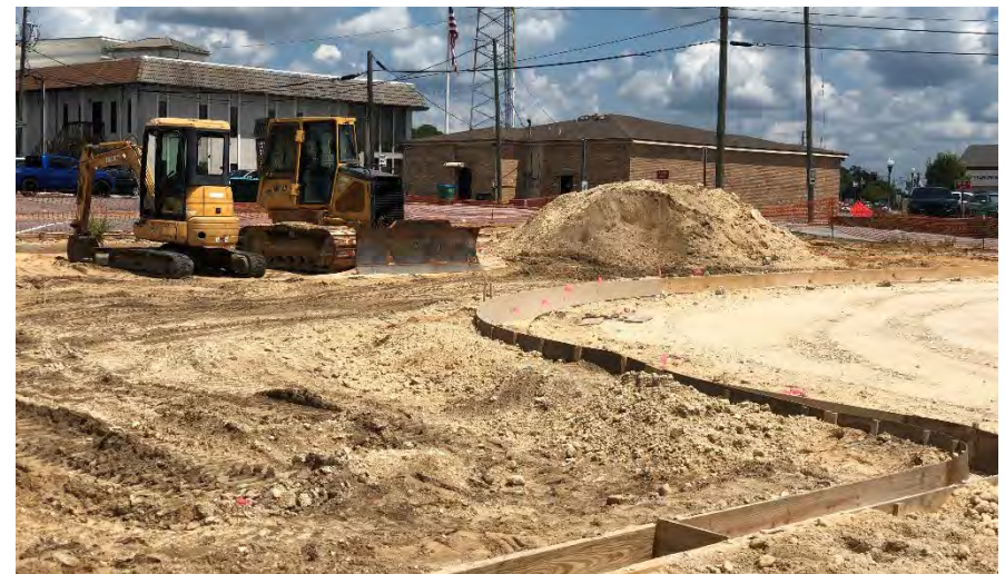
New parking lot being constructed at the southeast corner of Wilson Street and Beech Avenue.
